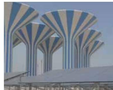
Desert-Specialized PV Module Bayan Water Tower Project, Kuwait
