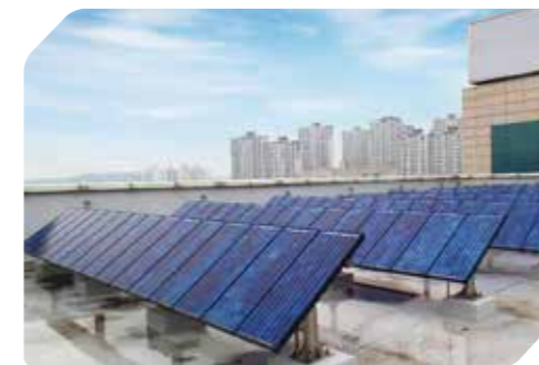
Test Site in Yongin-Si, GyeongGi-Do (March, 2020)
