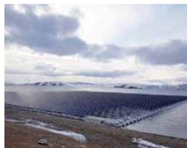
Water Floating PV Module Terhin Chagan Lake, Mongolia
